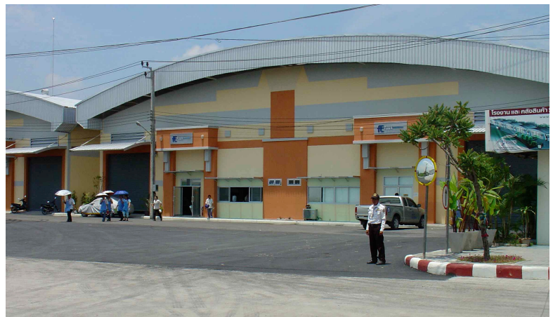
New Flux International Ltd. warehouse building – situated in connection to our manufacturing facilities.
